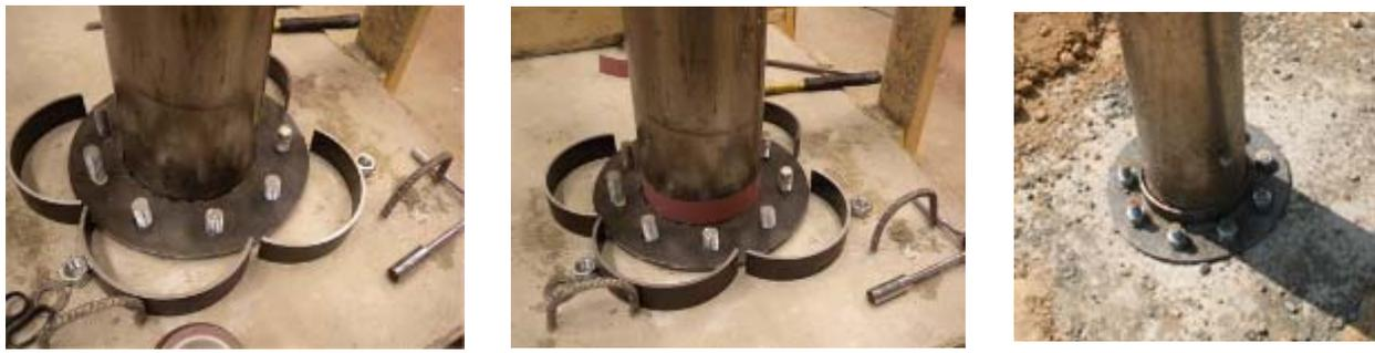
**Figure 2. Steel Collar: Components (Left and Middle) and Construction (Right)**
